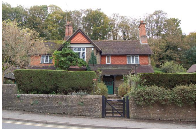
Figure 12: Greystones, Brighton Road.
