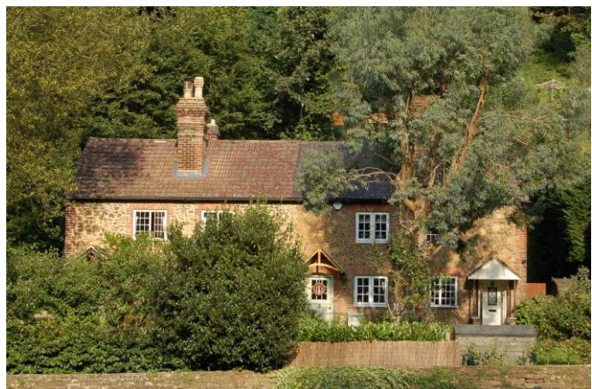
Figure 13: 103 and 105 Brighton Road
